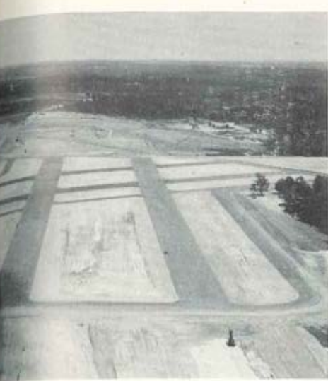
with 500-foot overruns on each end, 9,300 feet of taxiways, and a 17½-acre maintenance apron will meet the increasing fixed-wing training requirements at the Alabama facility. (U.S. Army photo).
