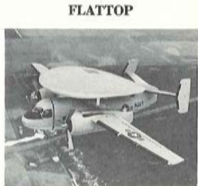
First flight of Grumman's WF-2 Tracer, a "saucer-topped" early warning airplane designed for Navy carrier operations, reveals the airplane's huge radome, largest yet designed for a carrier-based airplane. Look close. Single engine performance underway.
