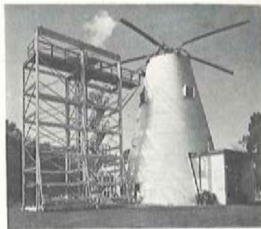
Overall view of new cone-shaped whirl test stand now in full operation at the Sikorsky Aircraft Division in Stratford, Conn. At left are the elevators used to carry personnel and huge rotor blades to the top of the stand.
