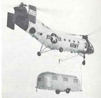
An H-21 Shawnee of the 80th Transportation Company (Lt Hel) is shown above lifting a 2,000 pound trailer during the testing of a new hoist on helicopters. The action took place at Bryant Airfield, Alaska, in preparation for Operation "Caribou Creek" participated in by men of the 503rd Airborne Infantry Regiment. (US Army photo/Jones).
