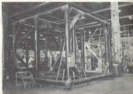
Aft Fuselage Main Assem- bly Fixture
