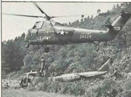
A CH-34 Choctaw helicopter of the 110th Aviation Company of the U.S. Army's Southern European Task Force (SETAF) begins a 14-mile flight from the Apennine foothills to an airfield in Sarzana, Italy. Its cargo is the fuselage of an Italian Army Model 204 helicopter that had suffered an engine failure. The recovery operation was performed jointly by members of the Italian Army's 2d Tactical Air Recon unit and SETAF's 17th Trans Det and 110th Aviation Co.
