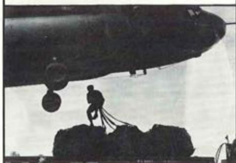
VUNG TAU, RVN - The 490th General Supply Company scores a Vietnam "1st" as it flies fresh vegetables in sling loads between land and ships at sea. The 3- to 4-ton loads are rigged into cargo nets for pickup by CH-47 Chinooks. Refrigerated ships speed the vegetables to US and Free World Forces in the Mekong Delta.
