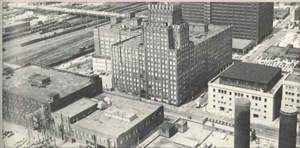
MART BUILDING, ST. LOUIS, MO.
